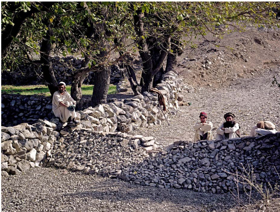
Figure 5. Example of an Afghanistan Check Dam (image by U. S. Army)
