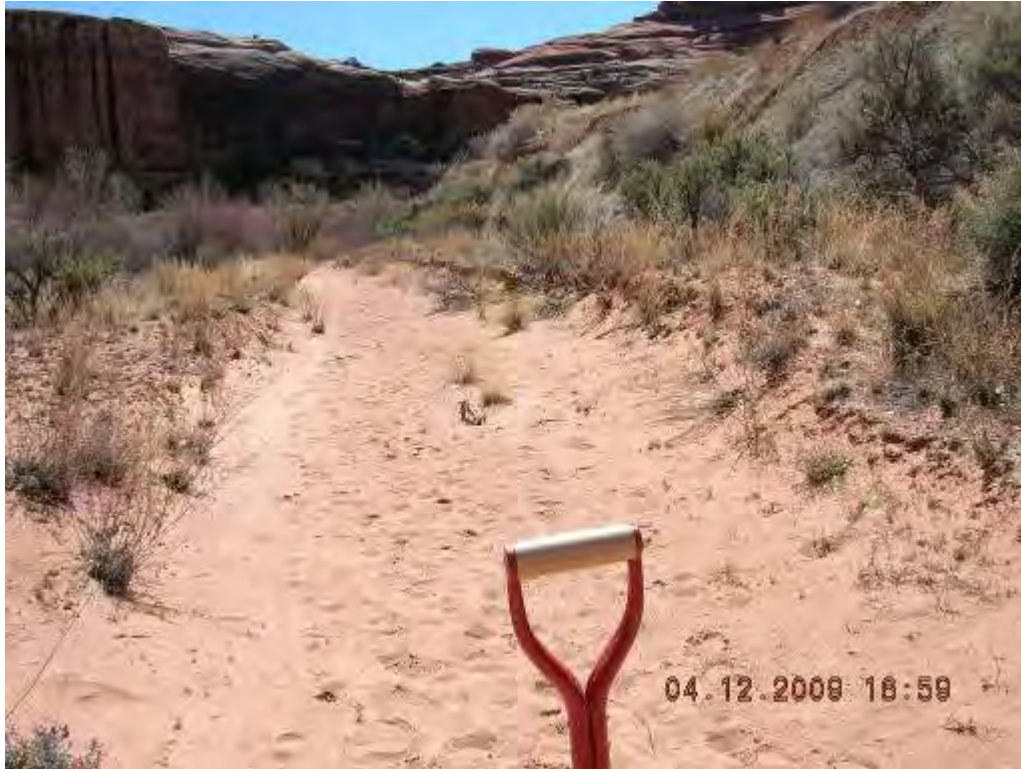
Natural sloughing and filling of unused road
