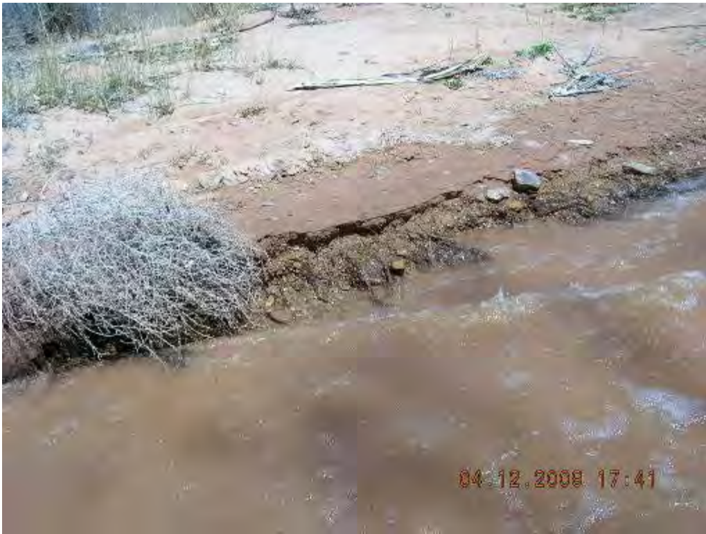
Erosion, turbidity, and root exposure from low velocity vehicle traverse
