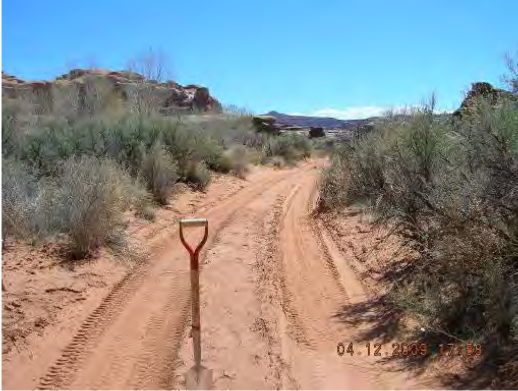
Erosion on Horse Canyon road on gently-sloping area
