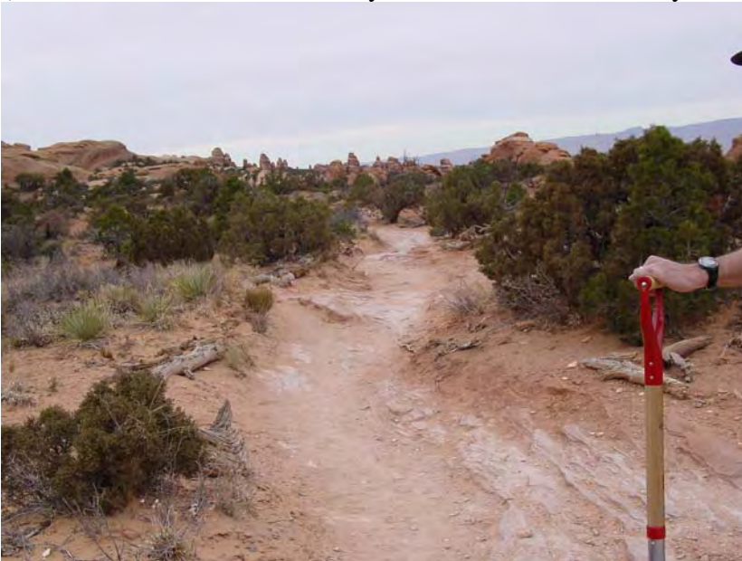
A trail rated in "Good" condition.
