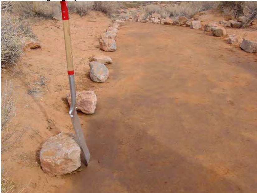
Chemical trail stabilization including rock borders.
