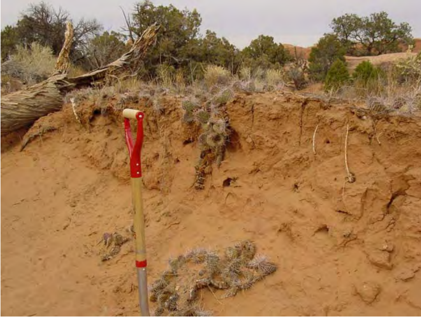
Active erosion, vegetation slough, and steep downcuts.
